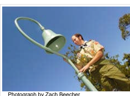
Photograph by Zach Beecher Boy Scout Brian Freund, with a little help from his friends, installed an El Camino Real bell at the east end of the Main Street bridge. The bell has been placed within 30 feet of where the actual section of the historic trail was located.
